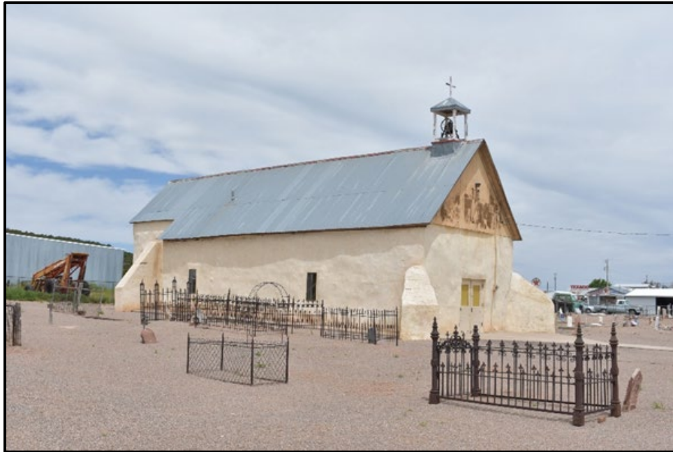
Figure 2.16. Adobe building with metal roof.
